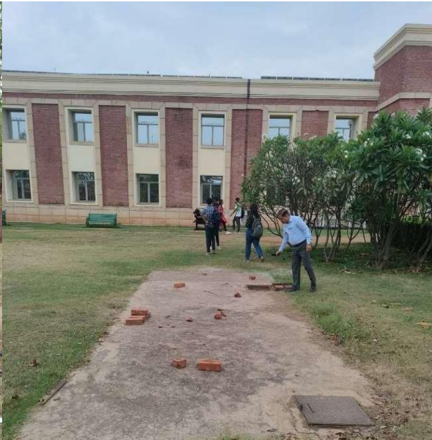
RWH Recharge Well
