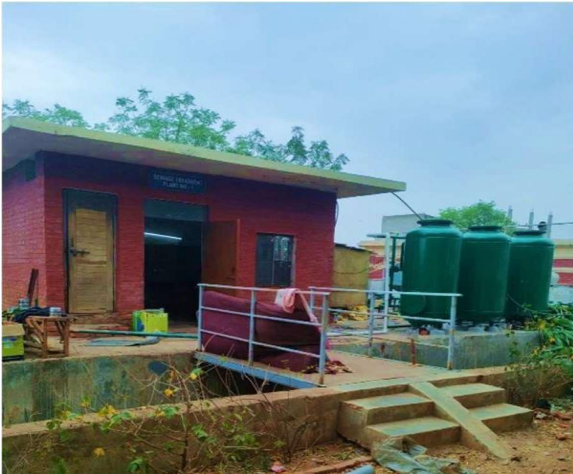
Sewage Treatment Plant
